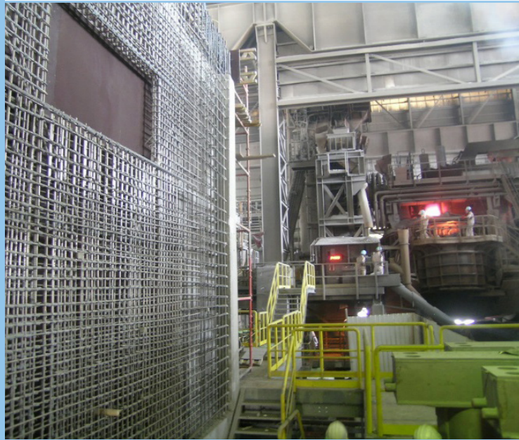
Melting Shop Building Extension, Italy
