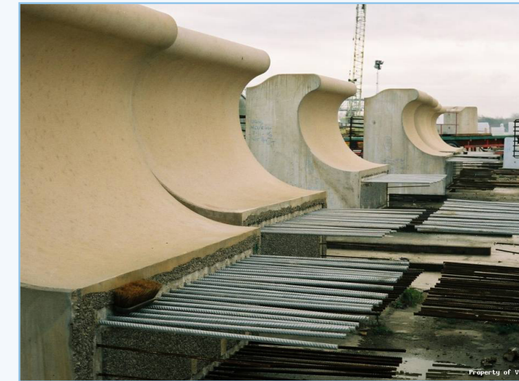
Left Picture: In-situ end wave wall unit
