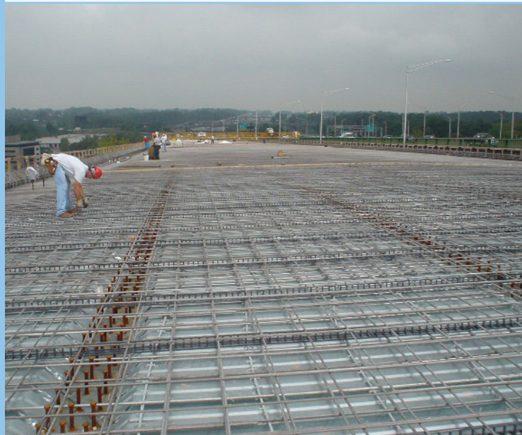
Bottom Picture: Dawlish Sea Defence repairs
