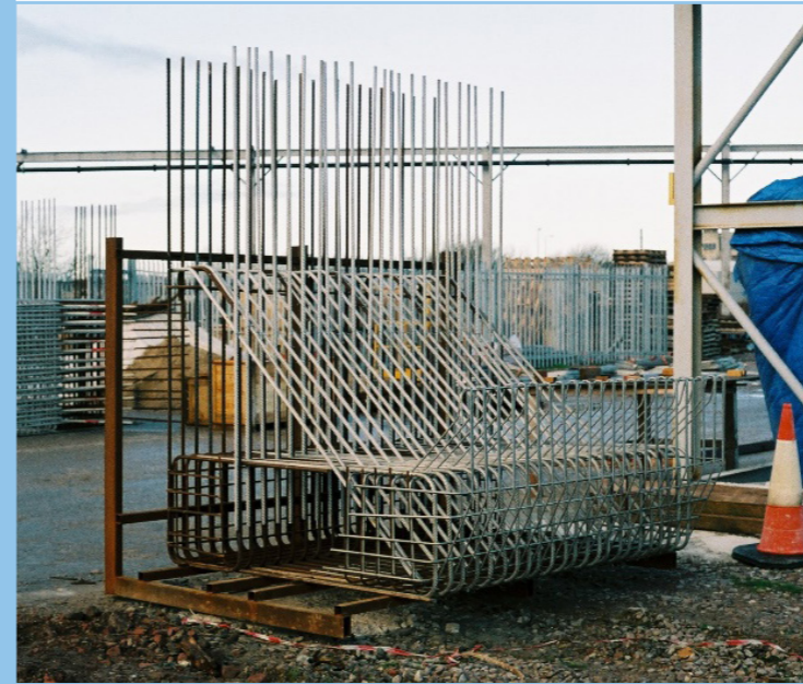
Top Picture: "naked" wave wall type 1 unit showing stainless steel used along side of carbon reinforcement.
