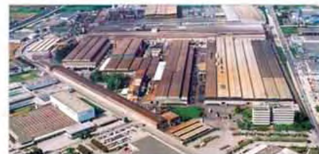
Vicenza plant, Italy (Total surface: 294.608 m 2 )
