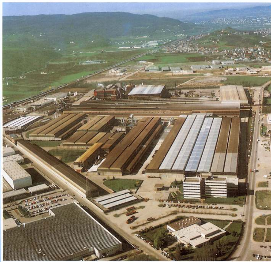
Aerial view of the Vicenza plant
